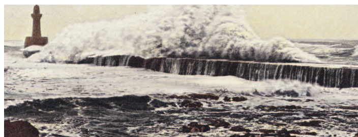
Cay's Breakwater still protects Aberdeen Harbour after 140 years Postcard 1910
