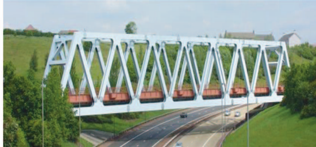
Fig. 5(c): A modern railway bridge consisting of triangulated frames
