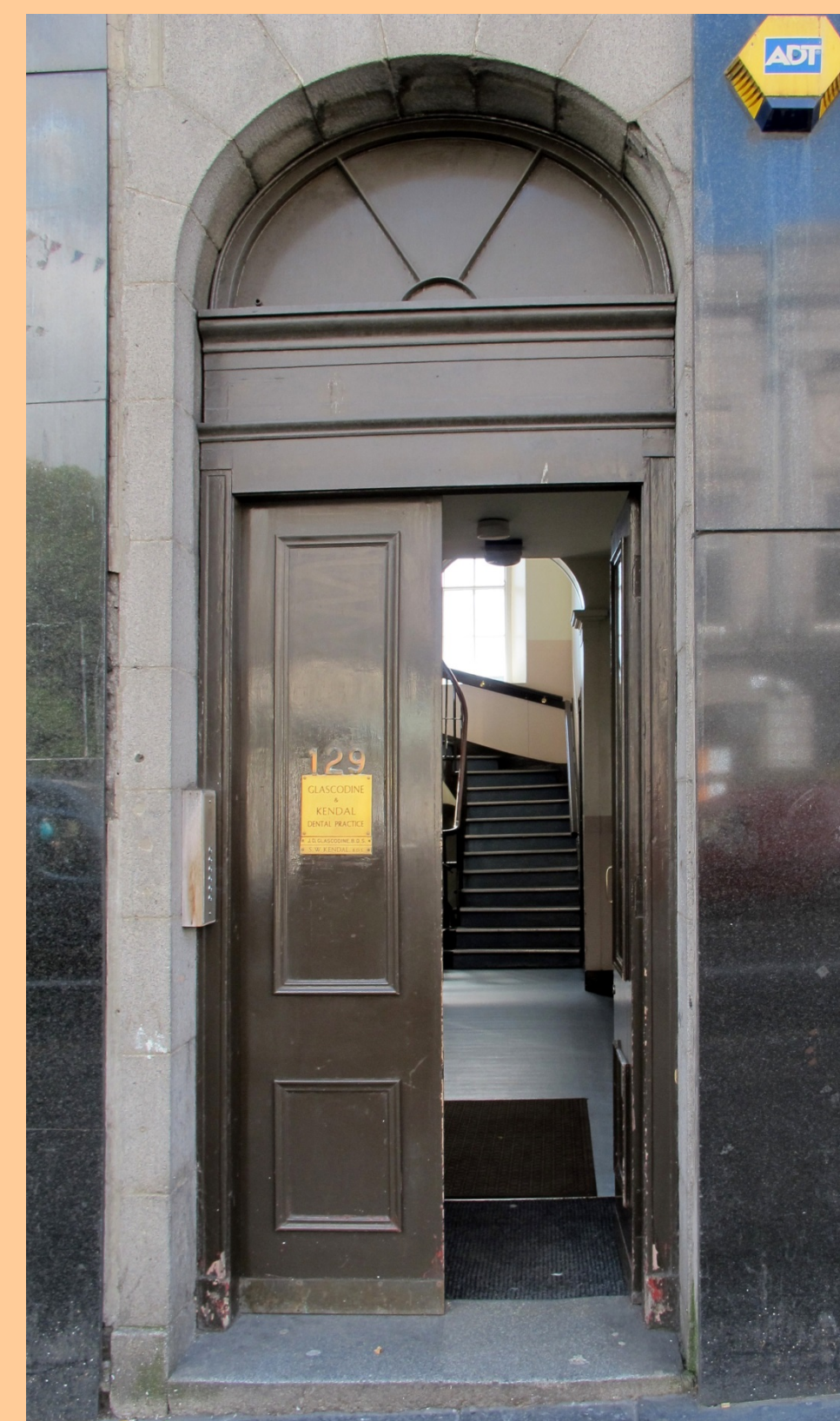
129 Union Street entrance
