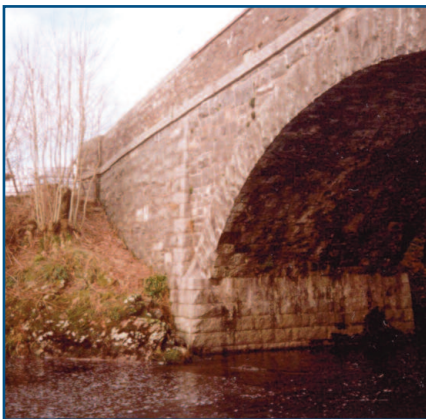
Cay's Glenlair road bridge – 45ft span © K. McCrae
