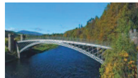
Fig. 1: Telford's Craigellachie Bridge
