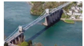
Fig. 2: Telford's Menai Suspension Bridge
